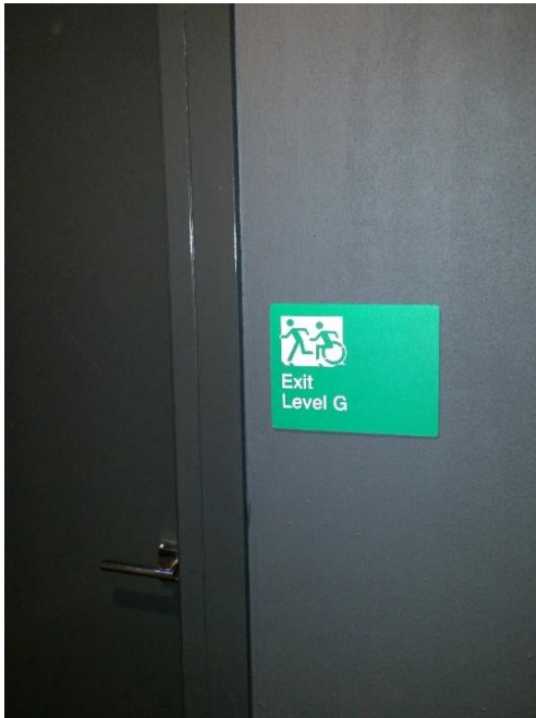
Figure 47: Photo of an Accessible Exit Sign installed on a Wall
